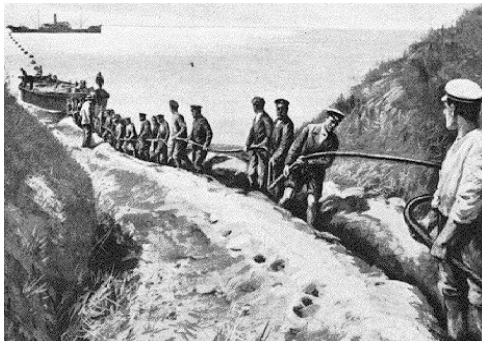
Submarine Cable Installation news sketch from the 1850's
